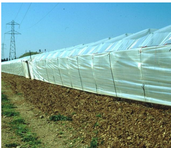
Fig. 3 – “Closed” plastic structure for “early covering” table grape vineyard (Apulia region, Southern Italy).
