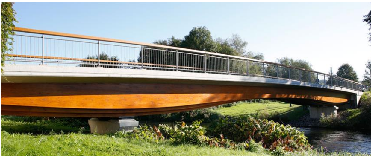
a) Most preko rijeke Ager u Lohmaru, Njemačka (izvor: https://www.ib-miebach.de/en/projects/timber-bridges/timber-concrete-composite-bridges/timber-concrete-composite-bridge-schiffarth-de.html )
