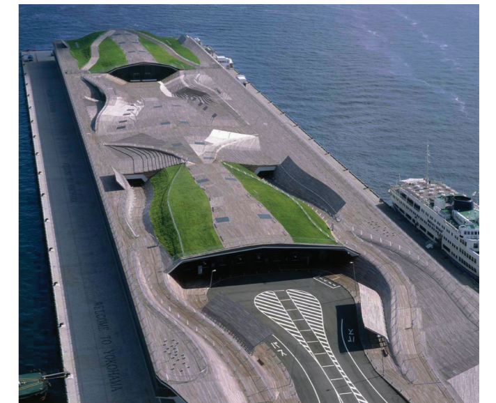
Yokohama Ferry Terminal_Foreign Office Architects
