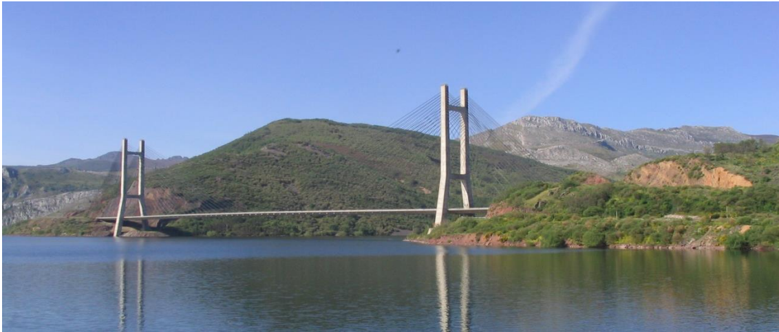
Figure 2.10 – Barrios De Luna Bridge ( http://www.arqueologiaypatrimonioindustrial.com/2007_07_01_archive.html , 2015)
