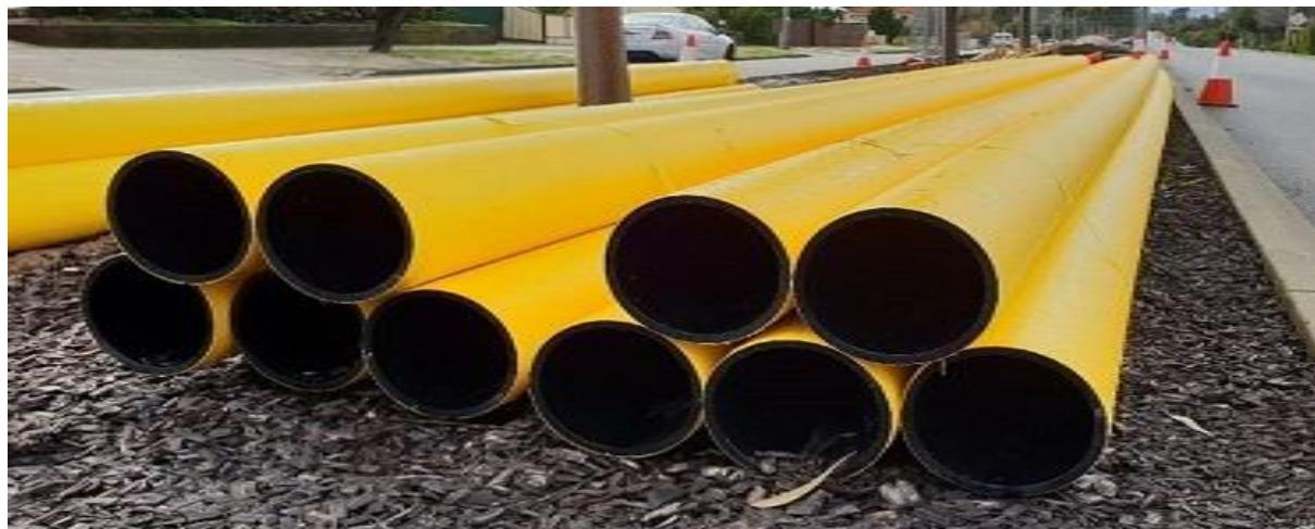
**Slika 2-1.** Polietilenske cijevi ([www.jamidarpipe.com](http://www.jamidarpipe.com), 2020)
