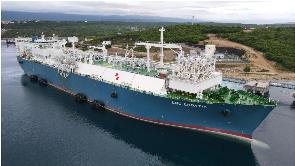
Figure 1-1 The Croatian LNG terminal (LNG Hrvatska, 2024)
