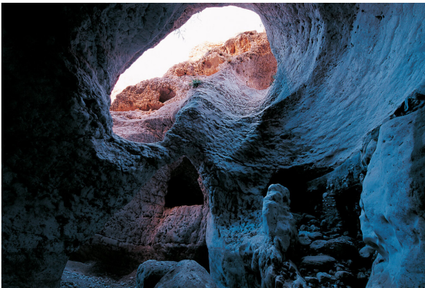
Image 20-21 Underground and surface manifestations of the Iranian qanat system used for water transportation and storage. In addition to providing water, qanats also help in cooling buildings and even preserving ice in some cases.
