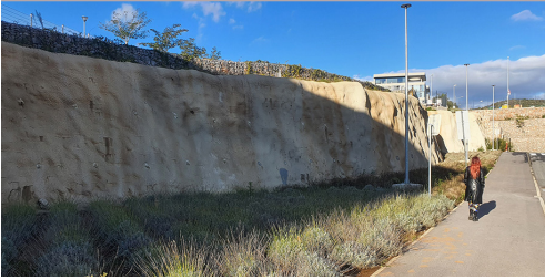
figure 45. - terrain disrupting horizontal connections between the hospital complex and the campus
