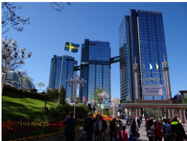
Slika 16. Hotel Gothia Towers
